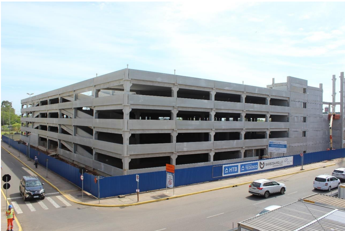
Image: New Parking Garage
