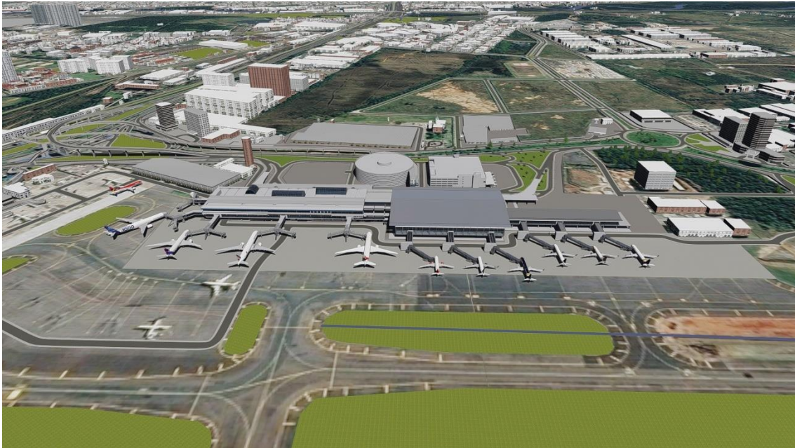
Image: New pier and passenger terminal 1 after expansion
